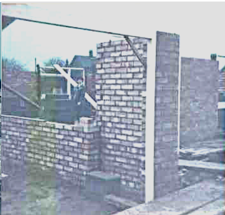
Construction of Number 55 on Plot number 510 -- February to June 1976
